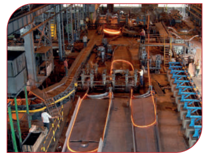
Jairaj Steel Plant Andhra Pradesh
